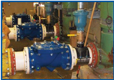
Swing-Flex® Check Valve with Backflow Actuator and Air Valve for Pump Discharge
