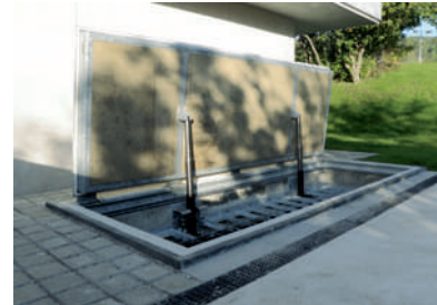
Hydraulic cover on a woodchip silo with a fire protection classification of F90 – Eisenstadt, Austria
