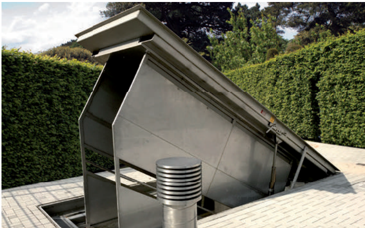
Pump station access – Seligenstadt
