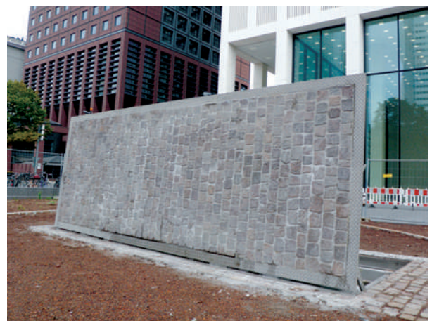
Escape hatch with paved cover – Frankfurt
