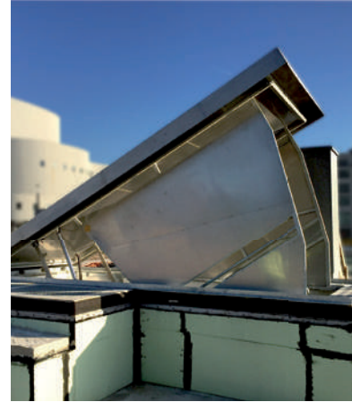
Hydraulic escape hatch cover – Düsseldorf
