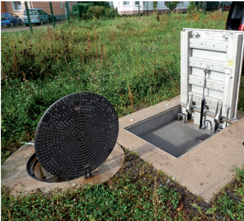
Combination: round cast-iron cover with hinge and an opening aid (on the left) and a stainless steel cover with an opening aid and safety grating (on the right)
