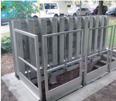
Three-piece cover with opening aid and folding guardrail – Frankfurt
