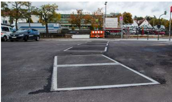
Backwater-proof covers filled with asphalt and with a load class of D400 – Ansbach
