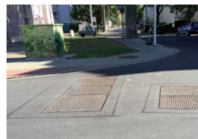
Series of cast-iron covers as a module cover and with a load class of D400 – Dresden
