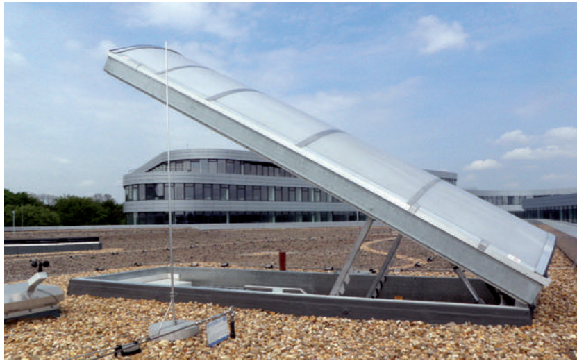
Hydraulic roof hatch and a damper for the smoke and heat venting system – Cologne
