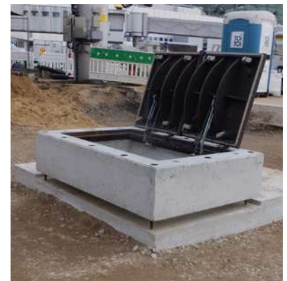
Prefabricated surface-water-tight cable shaft cover with a height-adjustable reinforced concrete frame – Düsseldorf
